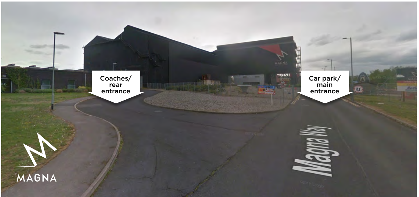
View from Manga Way/entrance to Magna. Coach parking is to the left, cars to the right.
